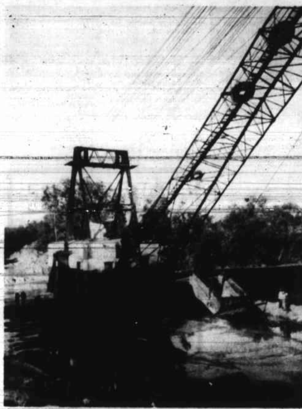
This huge 1,250,000 pound dragline, with 14 cubic yard bucket, was "walked" across the Colorado River last Thursday on route from Parker Bros. Eagle Lake gravel plant to the Altair plant, a distance of 6.5 miles.
